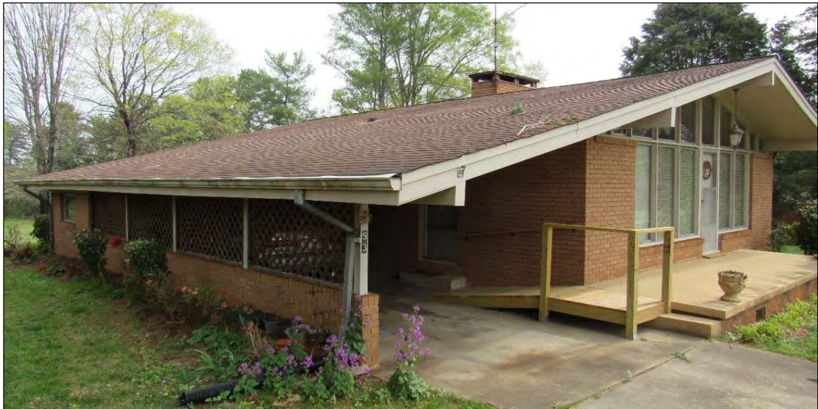
Photo 45: House, Carport Detail, Southwest Oblique.
