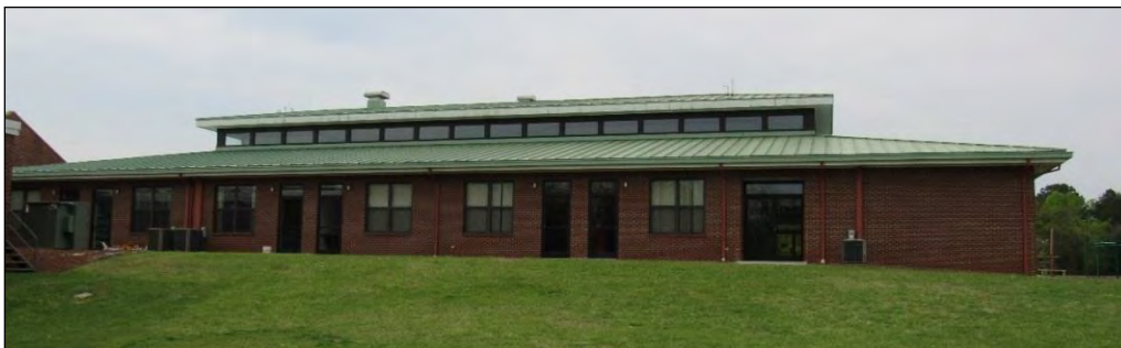
Photo 58: Circa 2000 Addition Detail, North Elevation.
