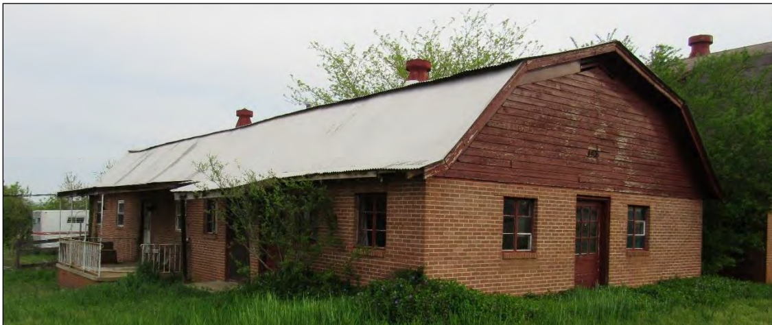
Photo 80: Office, South Oblique.
