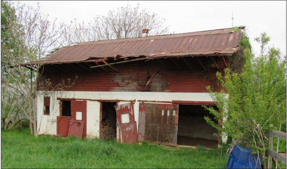
Photo 83: Barn, East Elevation.
