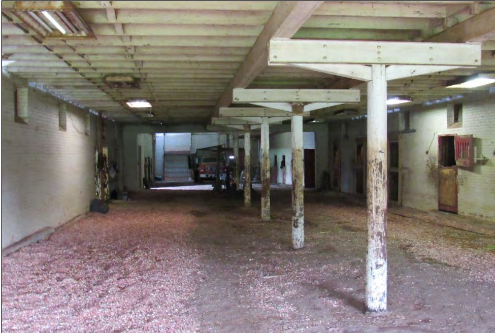
Photo 78: Interior of the Horse Barn, Looking Northwest.
