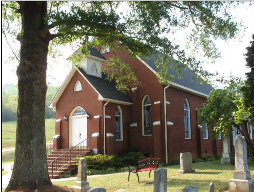
Photo 74: Mt. Olive Baptist Church, 210 Mt. Olive Church Road, Taylorsville, North Carolina.
