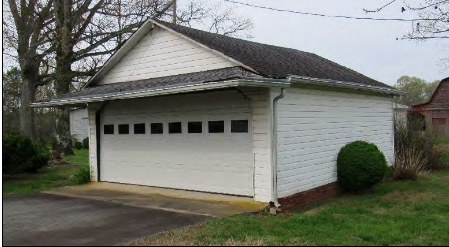
Photo 36: Garage, Northeast Oblique.
