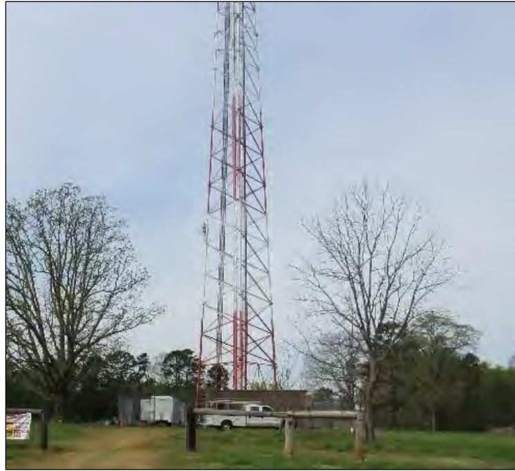
Photo 20: Cell Tower, Looking Southwest.
