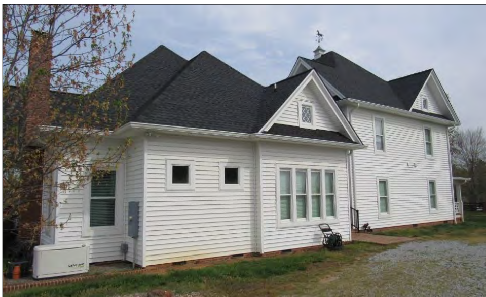
Photo 12: House, Addition Detail, Southeast Elevation.
