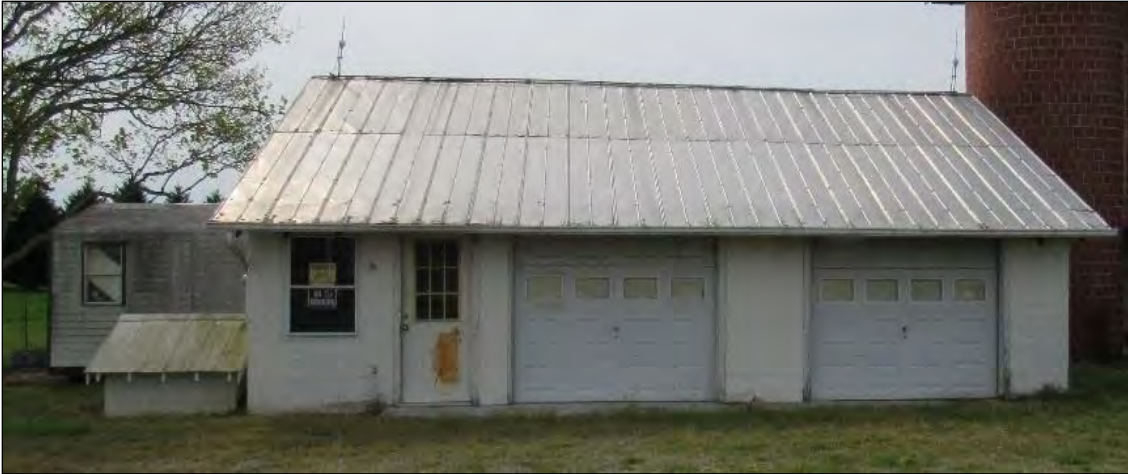
Photo 14: Garage, Northwest Elevation.
