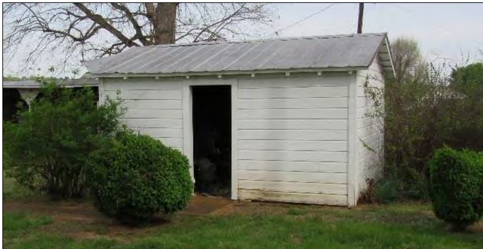
Photo 37: Shed, Southeast Oblique.
