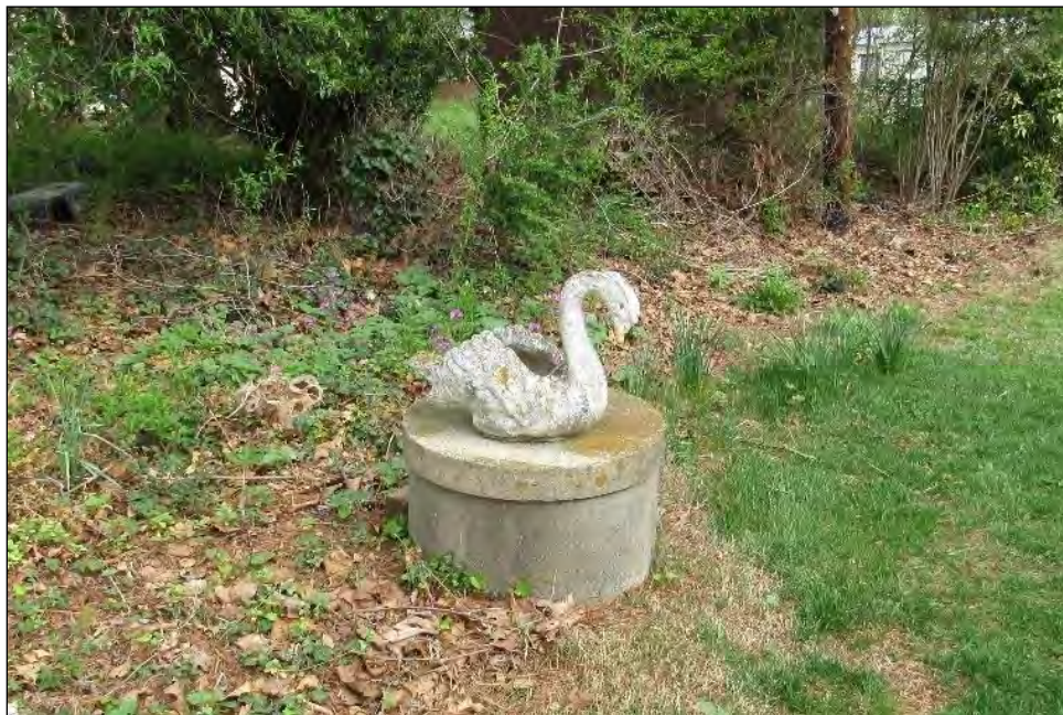
Photo 48: Well Cap, Looking North.
