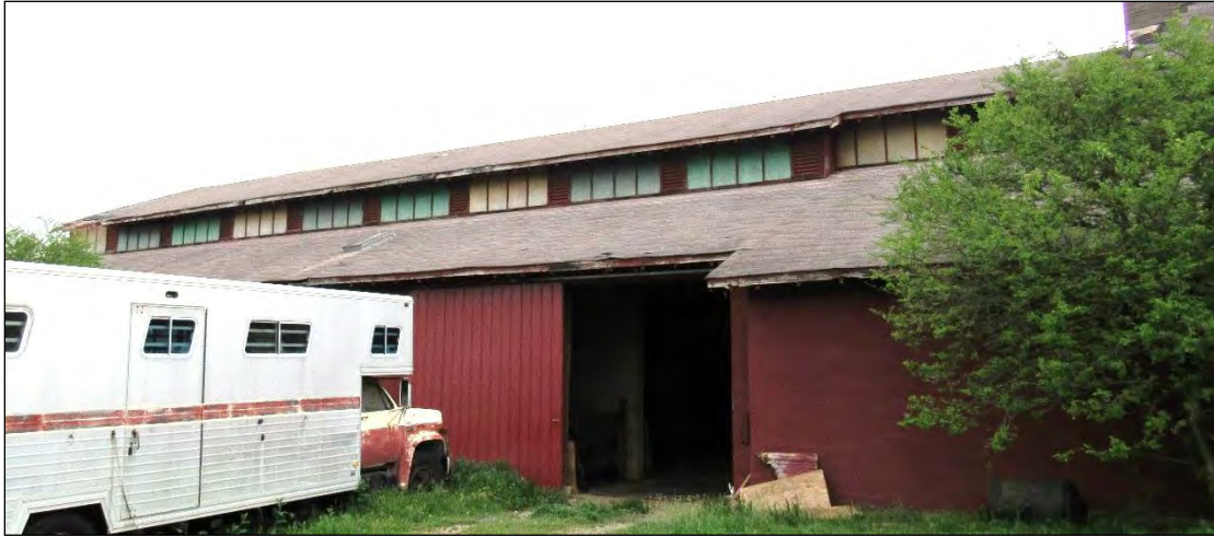
Photo 79: The Horsebarn LLC, Addition Detail, Southwest Elevation.
