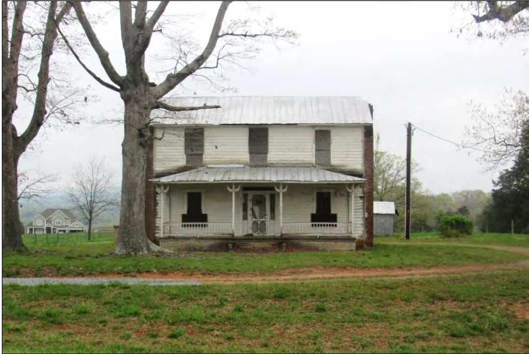
Photo 7: The D. P. Shufford House, 6108 West N.C. 10 Highway (CT0988).
