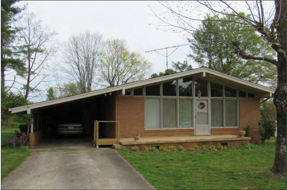
Photo 44: House, South Elevation.
