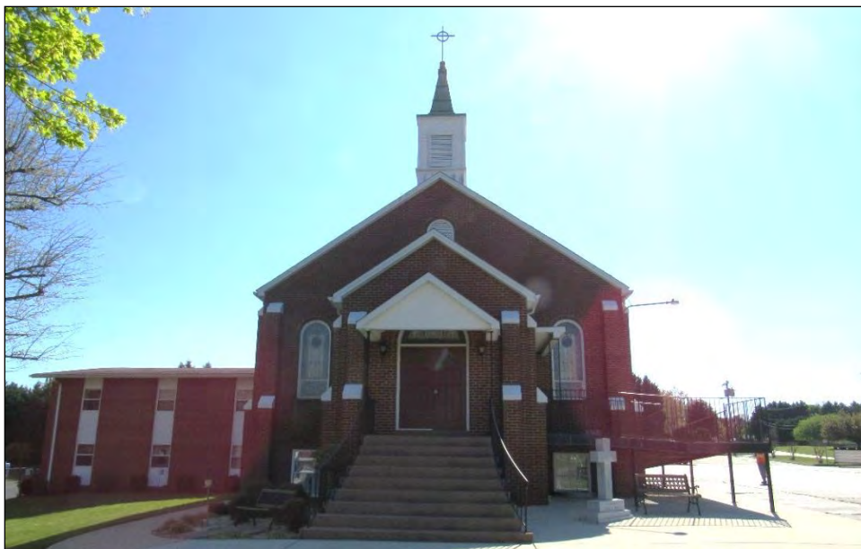
Photo 66: Church, Northeast (Primary) Elevation.
