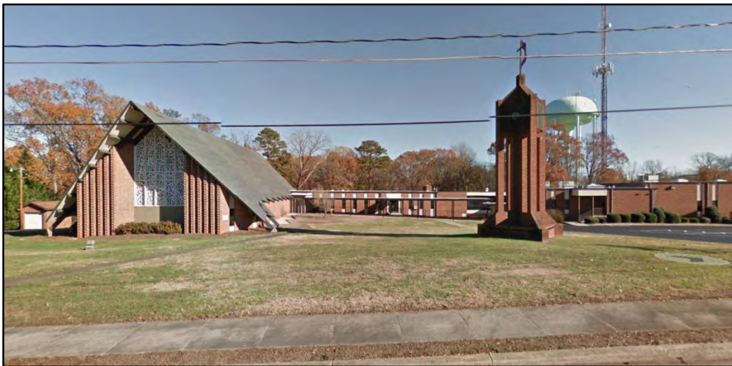
Photo 63: Highland Methodist Church (CT1367), 1020 12th Street Place NE, Hickory, North Carolina.
