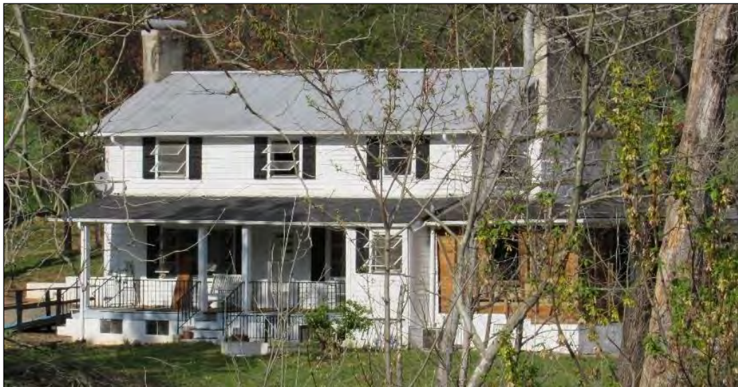
Photo 3: House at 7031 N.C. Highway 127, Addition Detail, Southwest Oblique.
