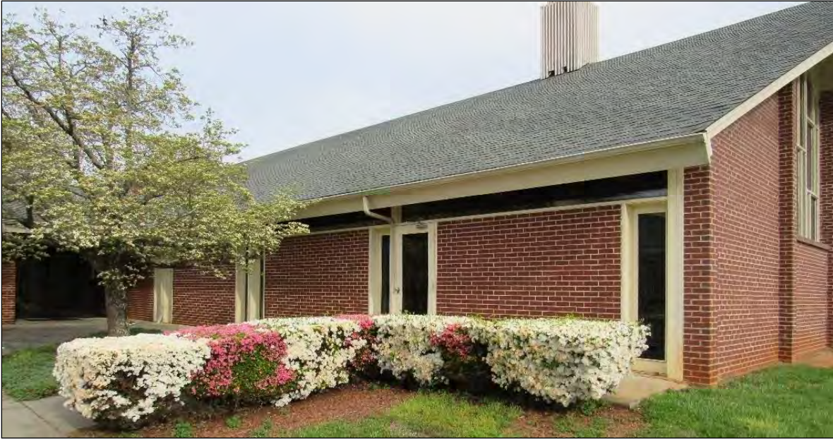
Photo 54: Church, View of South Elevation.
