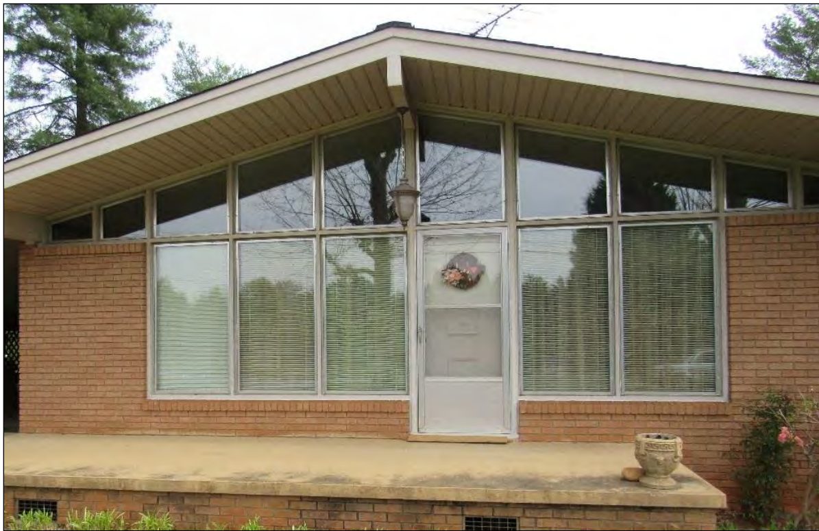
Photo 46: House, Window Detail, South Elevation.
