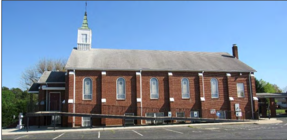
Photo 65: Shiloh Lutheran Church, Northwest Elevation.
