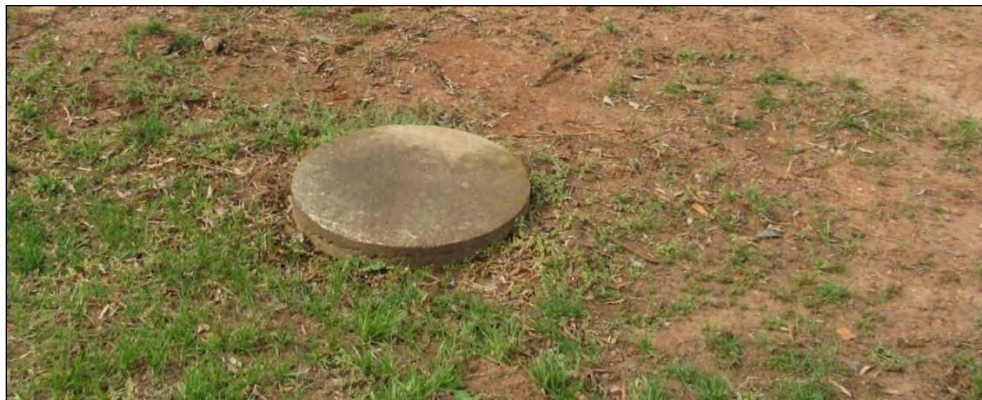
Photo 25: Well Cap, Looking South.
