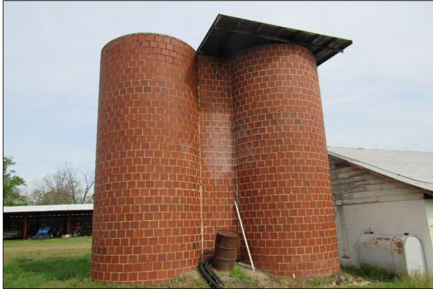
Photo 16: Silo Structure, Looking Northwest.
