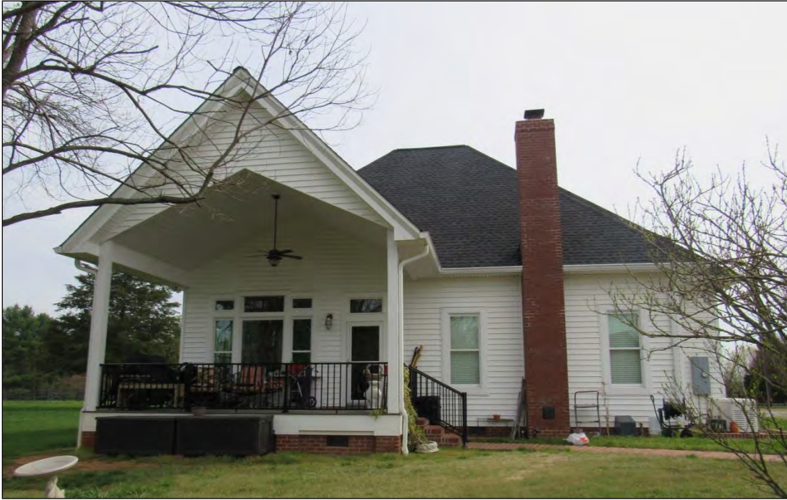
Photo 13: House, Addition Detail, Southwest Elevation.
