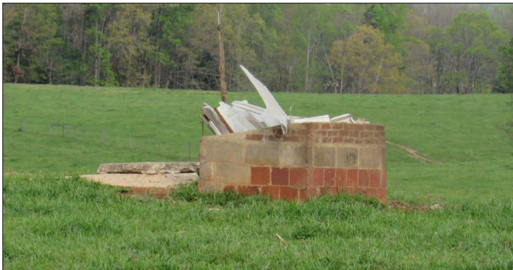
Photo 41: Foundation Remains, Looking North.
