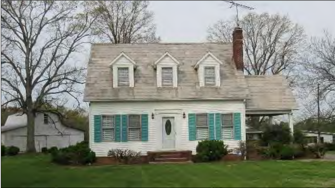
Photo 29: House, East Elevation.
