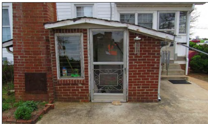
Photo 32: House, Addition Detail, West Elevation.
