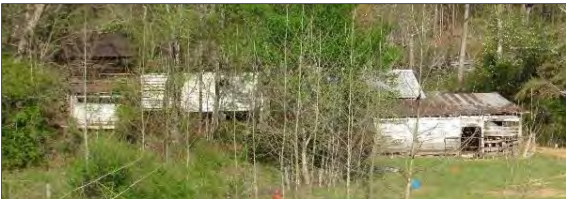
Photo 6: The Circa-1945 Barn (Left) and Circa-1940 Outbuilding (Right), Looking East.
