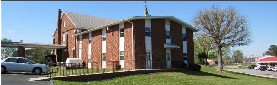
Photo 67: Church Addition South Oblique.
